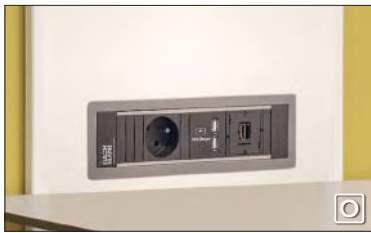
MEDIA PORT AND POWER SUPPLY 230 V
